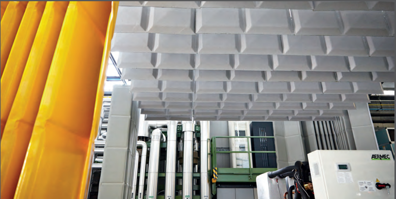
Test chamber for water-cooled units
