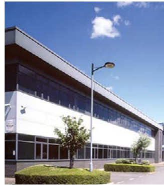
Redhill Data Centre. Redhill, Great Britain.
