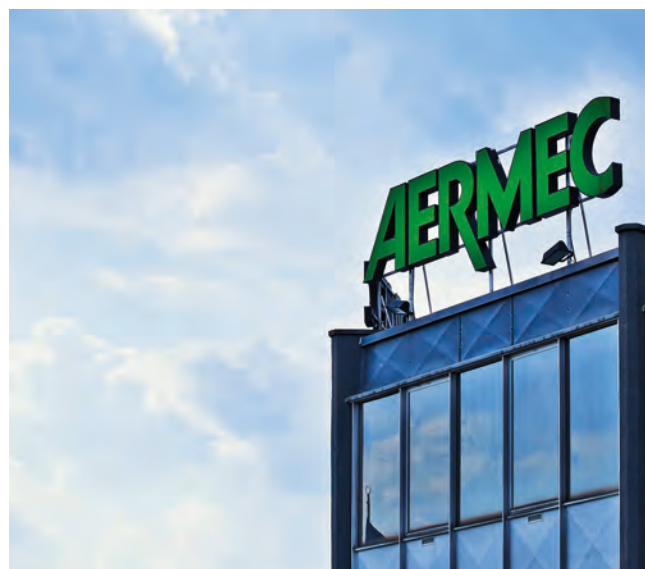
View from above of the factory and main entrance
